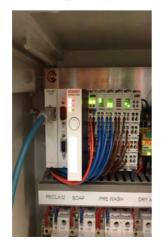
2.5K Control panel has only one control panel mounted on the machine and it has the digital display in lower part of the panel and no Ethernet cable.
